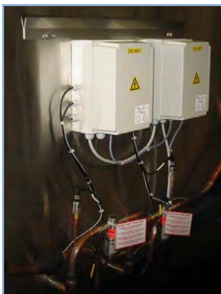
Eco-Tronic mounted on the tank and protected by a stainless steel hood
