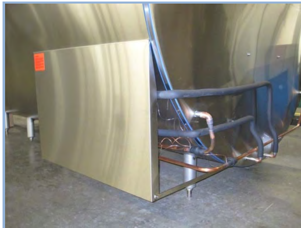
Example of bended cooling pipes on the right hand side
