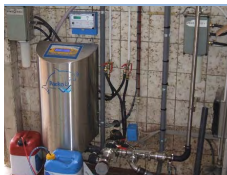
Example of an outdoors REM/DX milk cooling tank – control unit inside the dairy
